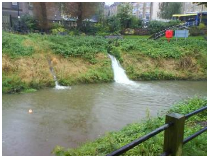
Figure 2 The river from the Market car park, showing the Chateau Gontier overflow in operation
