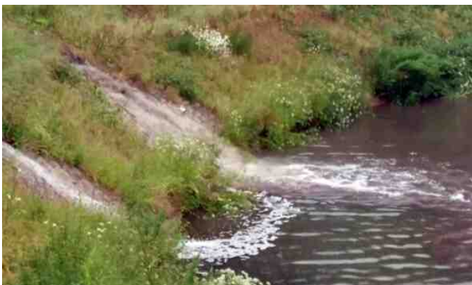
12 June: Sewage flowing into the river via the Market Place CSO. There were 130 hours of such spillages here in 2019
