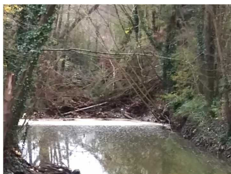
A serious blockage adjacent to Frome Sewage Treatment works off Weylands.
